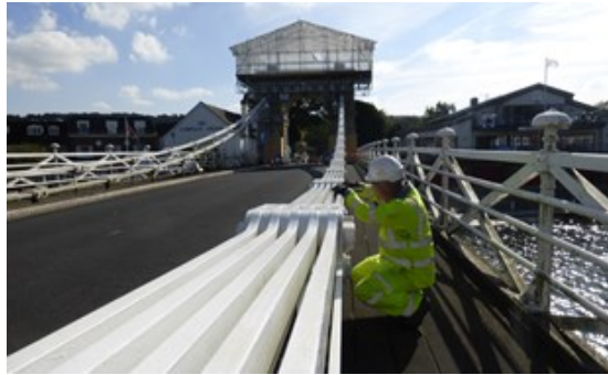
An engineer carries out stress-testing on Marlow Bridge during the two-month closure in the autumn
